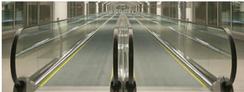
**Description:** A major manufacturer of moving walkways has developed an innovative high speed walkway that can transport up to 7,300 people per hour. The walkway is driven by smooth, compact Ramsey drive systems that provide normal walk way speeds at entrance and exit, while accelerating to higher speeds in central sections. Precise timing, smooth operation, and long life are important requirements in the application. The customer chose Ramsey chain and sprockets as the best solution.
